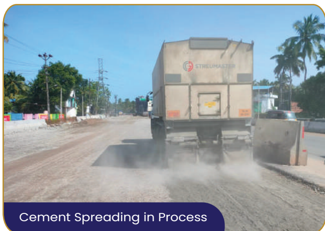
New CTB Layer Stabilization in Progress
