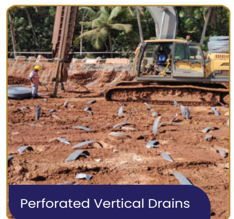
Retaining Wall Ground Improvement
