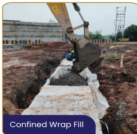
Retaining Wall Ground Improvement
